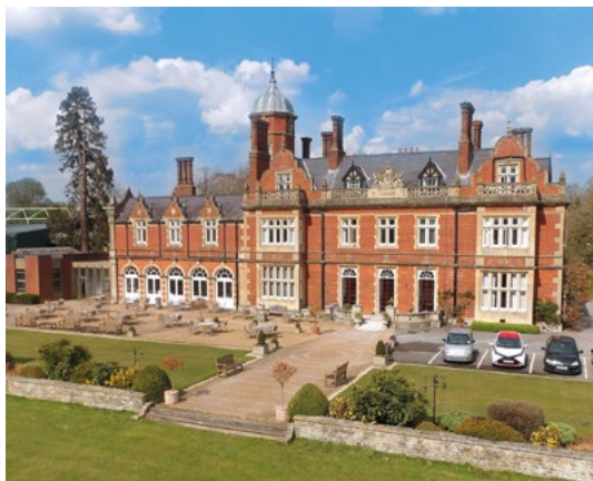
Howbery Park, QE head office location
